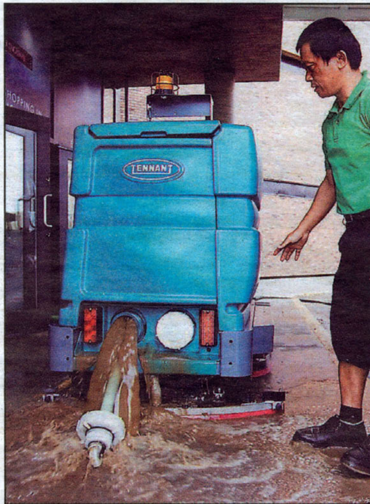
Cleanup is underway at Kingsway Garden Mall after a water main burst Friday afternoon.
